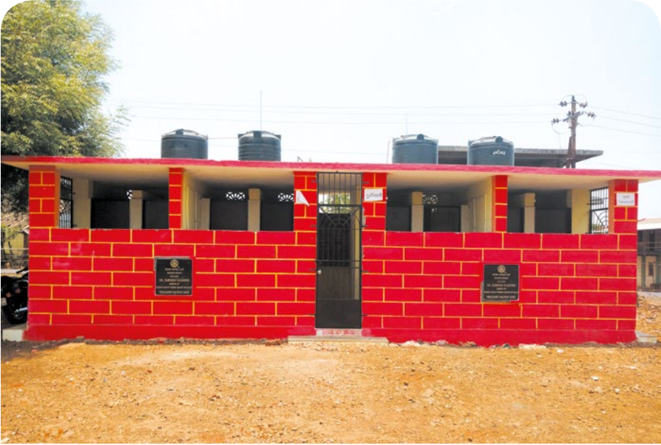
Rotary International, Sukhada Project, Thane, Maharashtra
